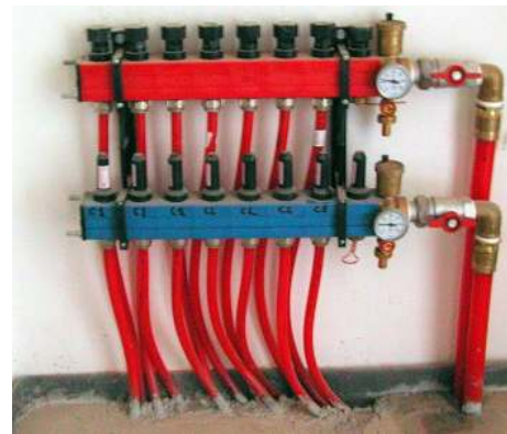
PEX piping. Photo: Chixoy
